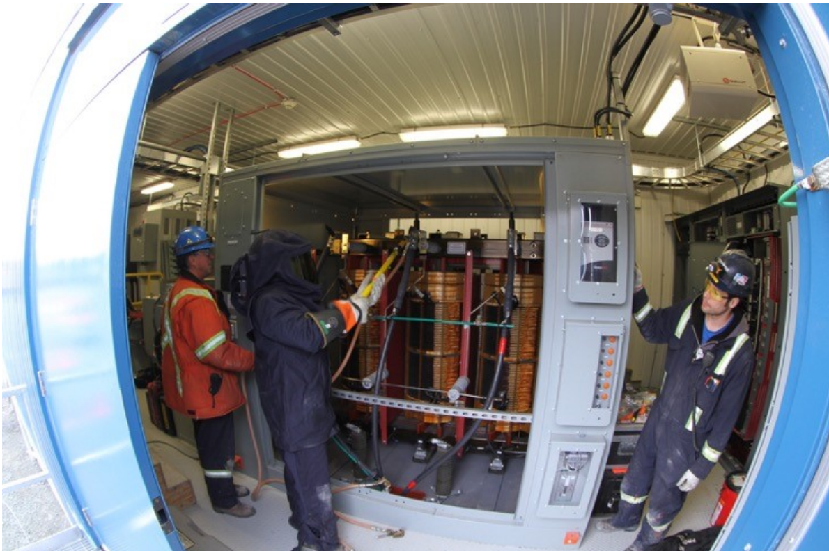
Figure 9 - Switchgear and Power Electronics Installation
